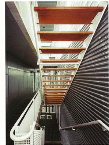
Trappenhuis met glazen lift. Stairtower with glass lift.
